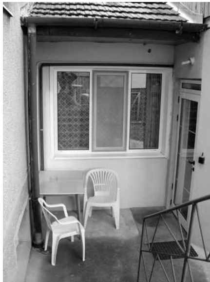
Picture 2. Wheelchair access
